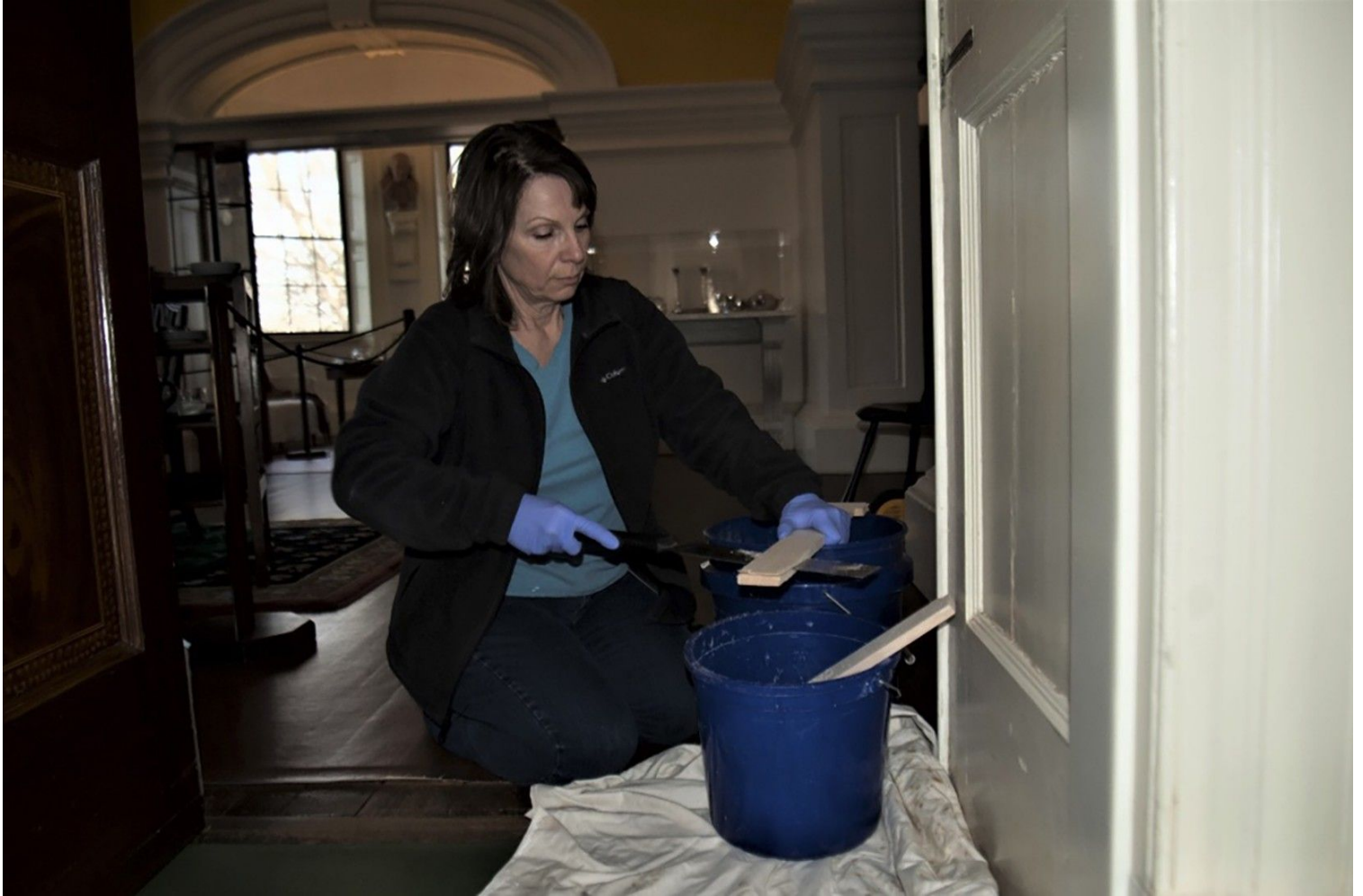
Restoration Specialist Carol Richardson cutting balsa wood to fill the wider portions of the crack.
