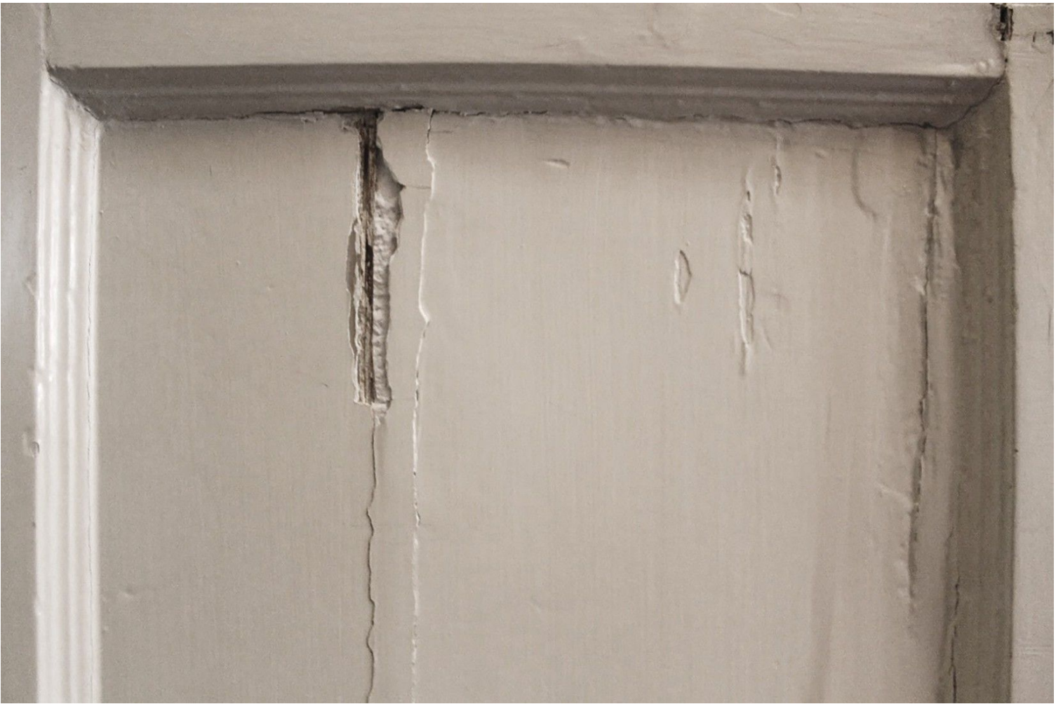
A previously filled crack in the door surround between the Parlor and Dining Room, before treatment.
